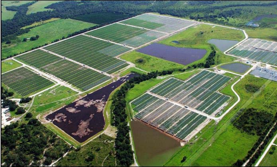
An aerial view of the Desoto Next Generation Solar Energy Center, the largest photovoltaic power plant in the nation. Newkirk Electric Associates, Muskegon, was heavily involved in its construction. It's being visited today by President Barack Obama.
