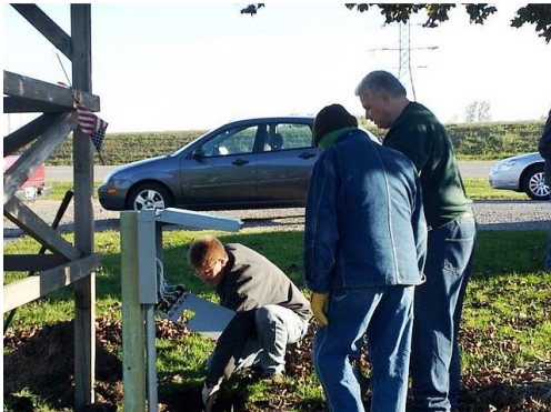
From left to right, apprentices Jason Lowe and Bill Chappell work with Training Director Dave Kitchen on installing an electrical pedestal at Muskegon's Veterans Memorial Park.
